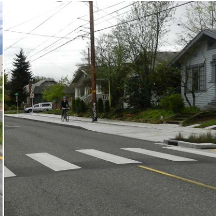
Sidepath Connecting Offset T-Intersections
