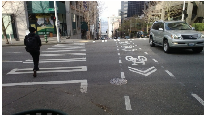
Shared lane markings and dashed lines are used to guide bicyclists through the intersection
