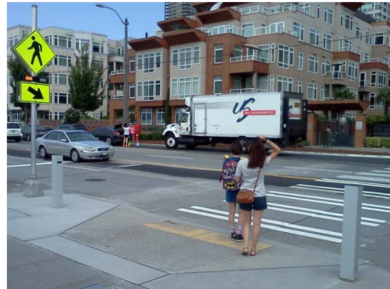
Rapid Flashing Beacon
