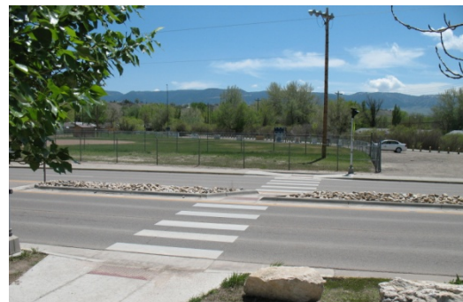
Crossing island on 13 th St
